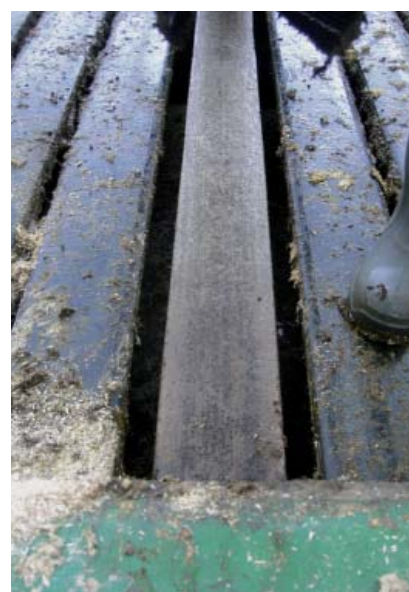
Picture 3: No accumulation of urine or faeces on the slat or beam under the Comfort Slat Mat
